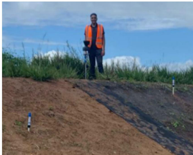
Installing vetiver grass to stabilize this hillside and protect against soil erosion and improve the quality of the soil
