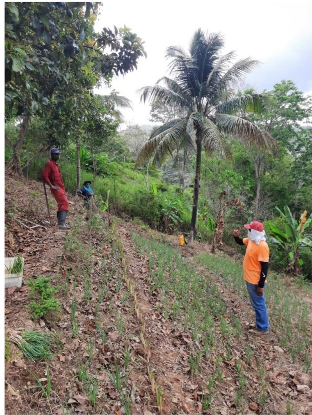
Installing vetiver grass to stabilize this hillside and protect against soil erosion and improve the quality of the soil
